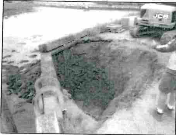
Photo 4.2-1: Excavation at the northeast end of the bulkhead.
