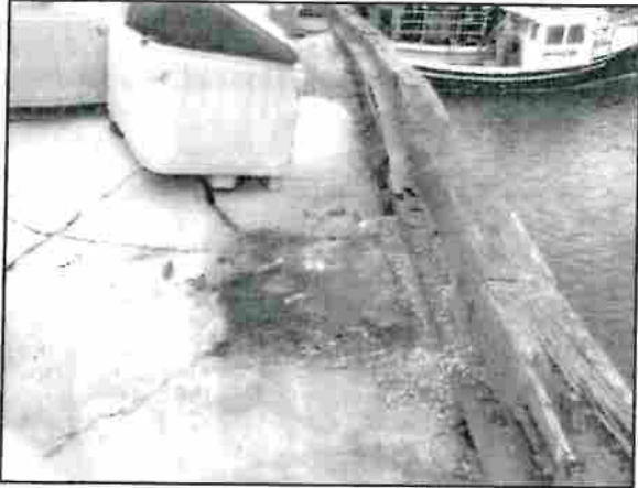
Photo 4.1-13: Removal of existing jib crane within the area of deterioration.
