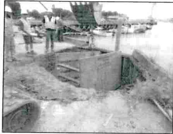
Photo 4.2-2: Placement of trench box.
