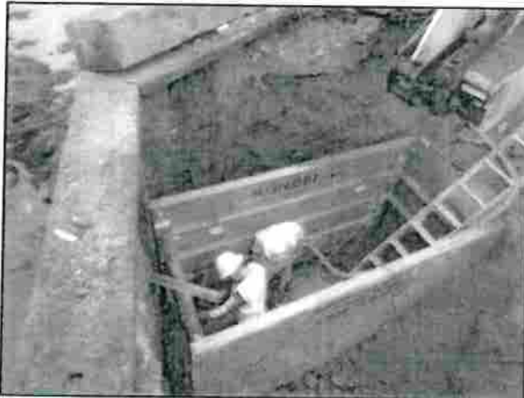
Photo 4.2-3: Additional excavation to expose the buried tieback system.
